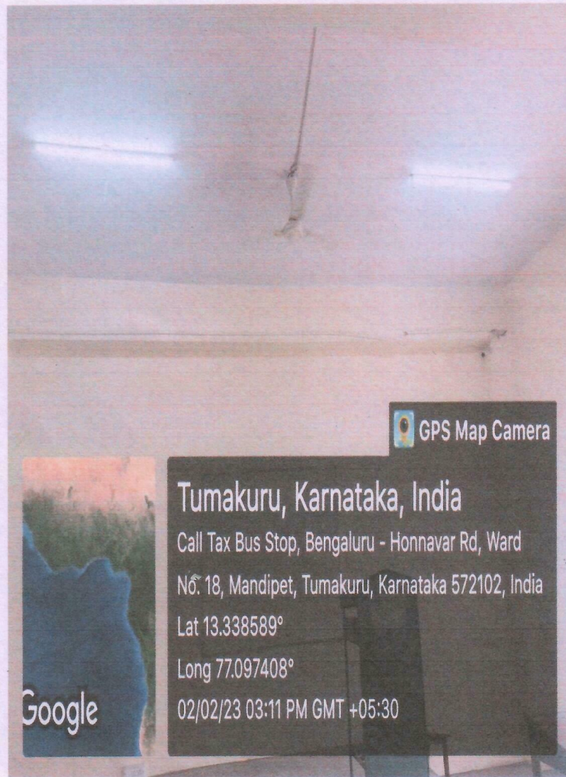
Photo of LED Tube Lights in Class Room
